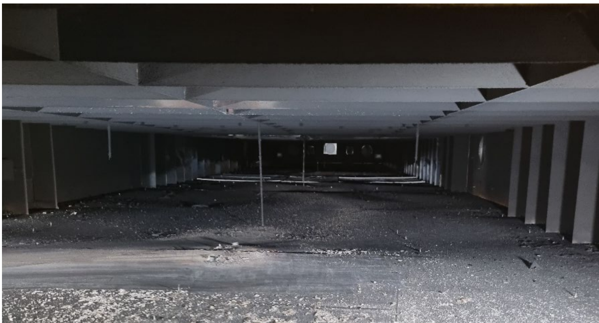
Figure 18: Photo from inside model. Beams are visible on side and in deckhead.
