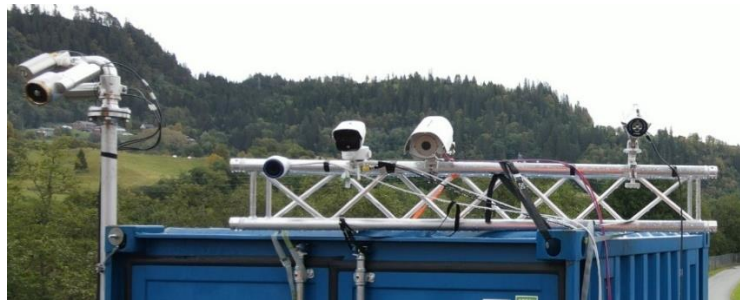
Figure 45: Detection sensors installed at the height of 7 m beside one of the fire monitors during the large-scale fire suppression tests. The sensors include thermal imaging and regular video cameras, as well as a triple-IR flame wavelength detector.
