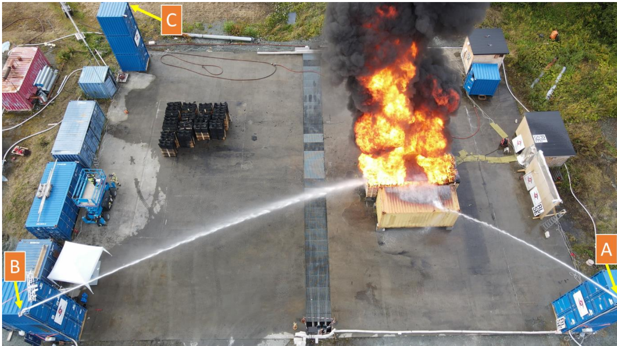
Figure 29: Photo showing the moment of activation of two of the three fire monitors (marked as A, B, and C) during a late-suppression scenario (300-s waiting time).
