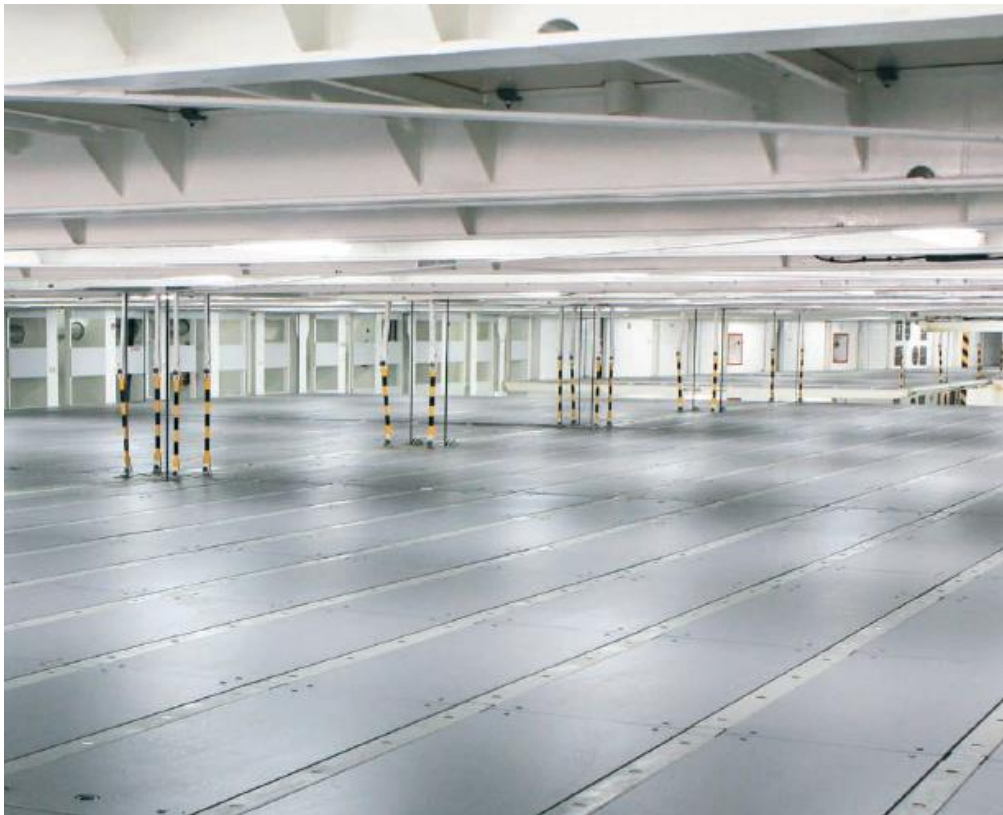
Figure 15. Plywood car deck panels
