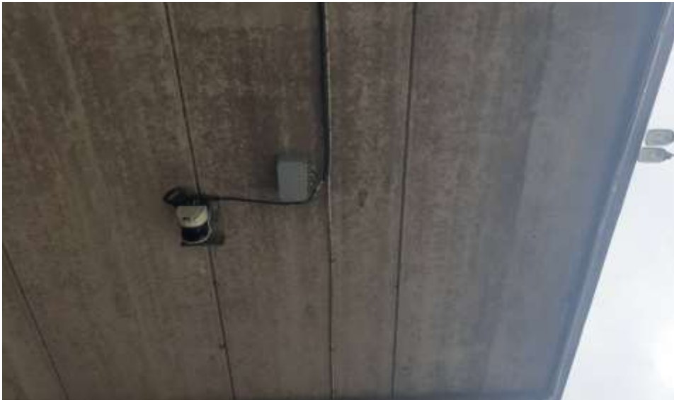
Figure 14 Forward positioning LiDAR at Majnabbe. (STL)
