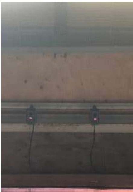
Figure 5 The ANPR cameras reading the rear of the vehicle. (STL)
