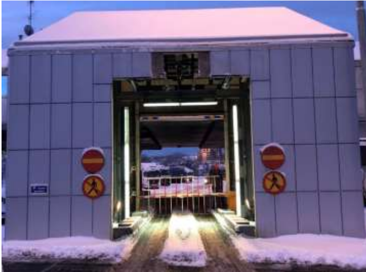
Figure 23 Exit of gate house after modification. (STL)
