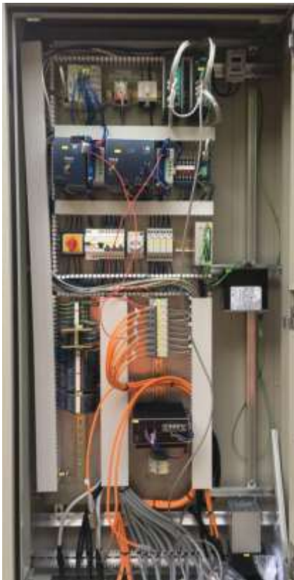
Figure 19 Interior of an VHD Cabinet. (SICK)
