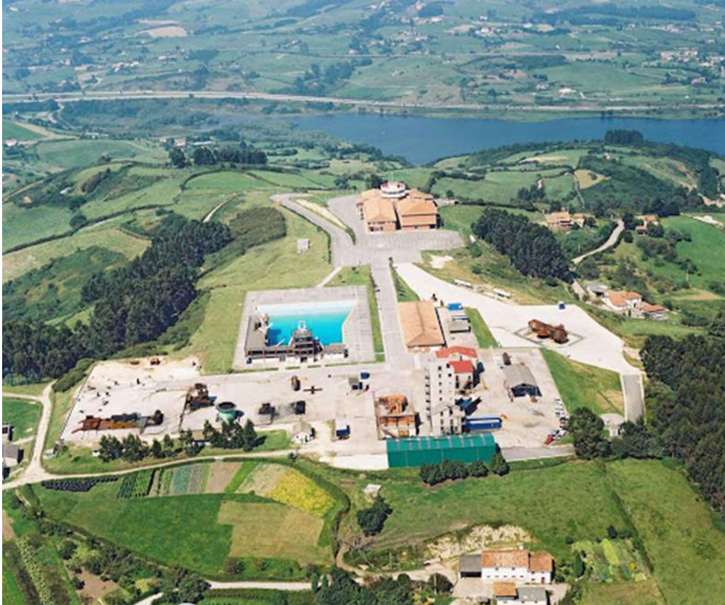
Figure 7 Jovellanos Safety Training Centre. Gijon Maritime Rescue Coordinator Centre. Aerial picture
