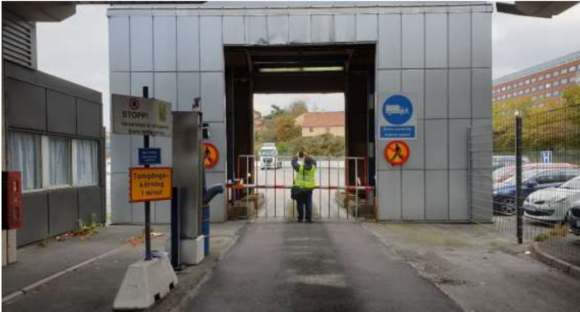
Figure 4 Gate and building at Majnabbe. (RISE)
