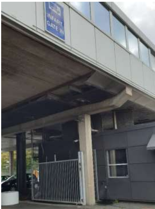
Figure 5 Front edge of office building in front of the gate. (RISE)
