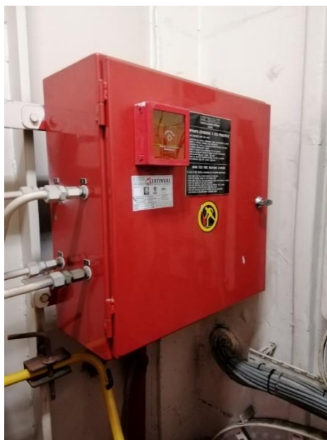
Figure 13. Release box for control of activation of the CO 2 system.
